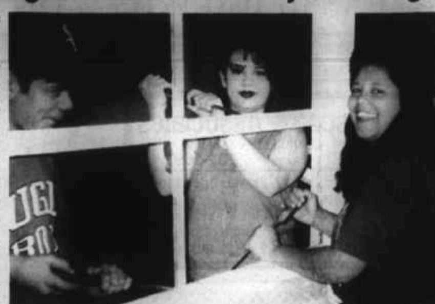
AISHA volunteers, pictured above, Ralph Castillo, Griselda Montalvo and Angie Castillo help replace and repair windows at the E.H. Henry Center.
